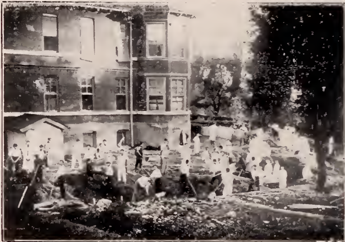
Students Volunteering to dig the foundations for an additional building.
